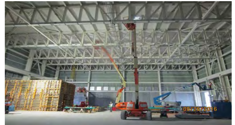
Installation of Lighting
