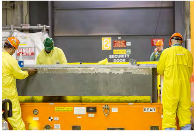
Vault Prep - Installation of Bulkheads
