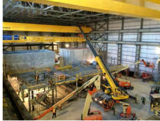
Installation of Waste Tooling System Platform
