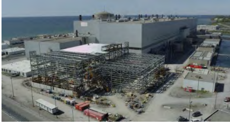
Erection of Structural Steel
