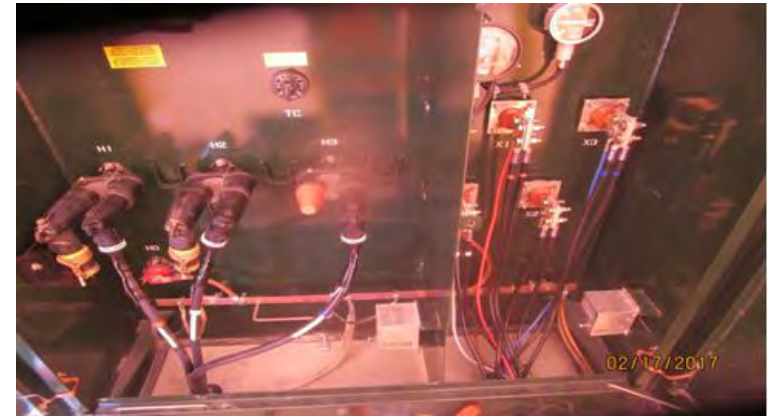
T20 Line and Load Terminations
