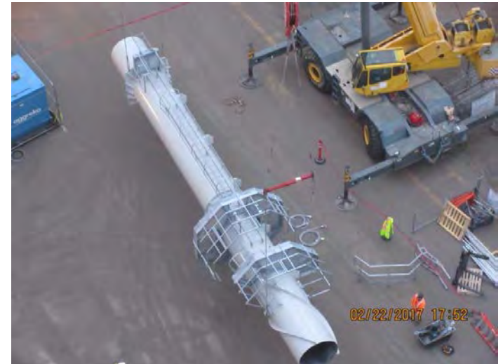
Installation of Landing Scrubber Stack
