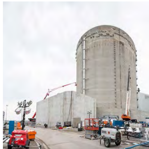
Installation of Exhaust Stack
