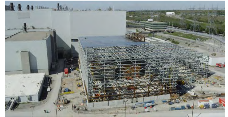
Structural Steel Installation
