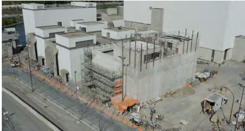
Completion of Civil Work
