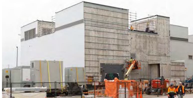
Installation of External Cladding
