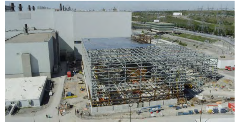
Erection of Structural Steel
