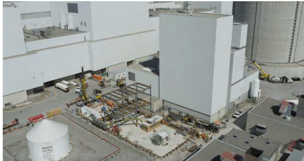
Erection of Structural Steel
