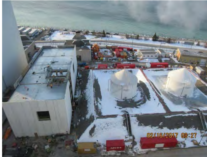
Completion of Building Envelope
